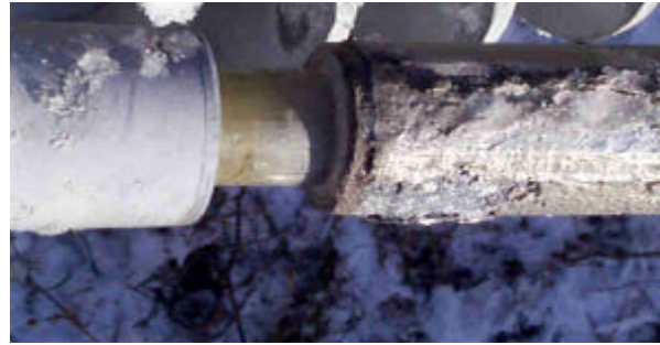
Fig. 4.2-2 : no damage after more than 10 years in service with an exposed FRP rod.
